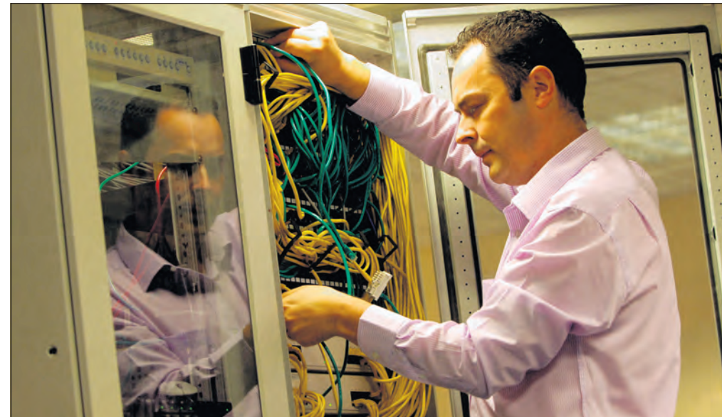
KEY PLAYER: Projects manager Alan Hill patching telephones and computers in on a network
